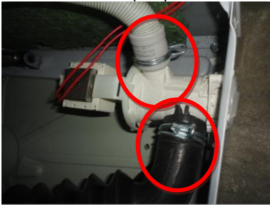
Picture 5.32 Drain pump Attachment/Detachment
