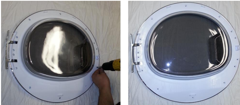
Figure 13.19. Unscrewing the rear plastic door
