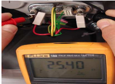
PICTURE E2-4: One of the cables on the heater is removed (left) and heater resistance
