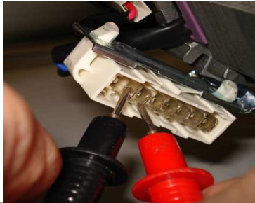
PICTURE 11-4: Motor coil resistance is being measured over the 8-pin motor.
