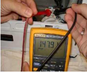
PICTURE E5-2: pump resistance is being measured over the pump connector
