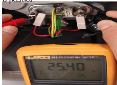
PICTURE E2-4: One of the cables on the heater is removed (left) and heater resistance is measured.
