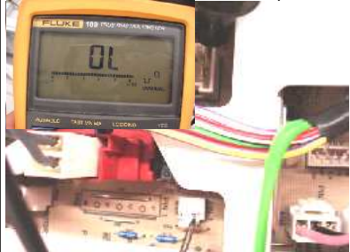
PICTURE E2-3: Short circuit check is being made between KN8-1 pin and KN5-1 pin.
