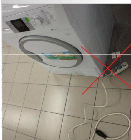
Inappropriate Extension Cable Usage
